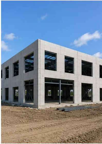
Ảnh số9. Structural frame completed according to project schedule
