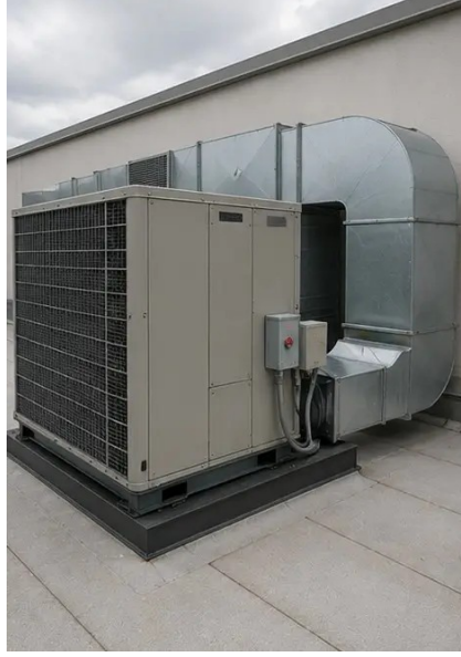
Photo #11. HVAC equipment condition assessed
