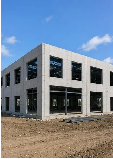
รูปภาพ №9. Structural frame completed according to project schedule
