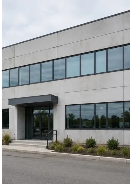
Photo #2. Framsidans fasadskick under besiktning
