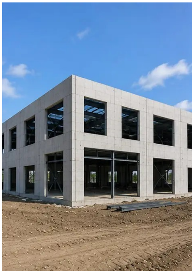
Foto Nr.9. Structural frame completed according to project schedule
