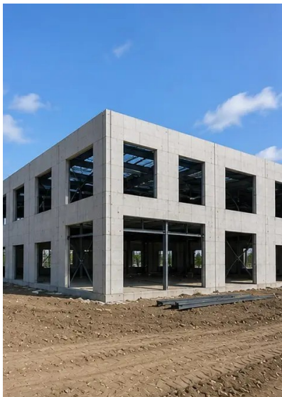
Foto št.9. Structural frame completed according to project schedule
