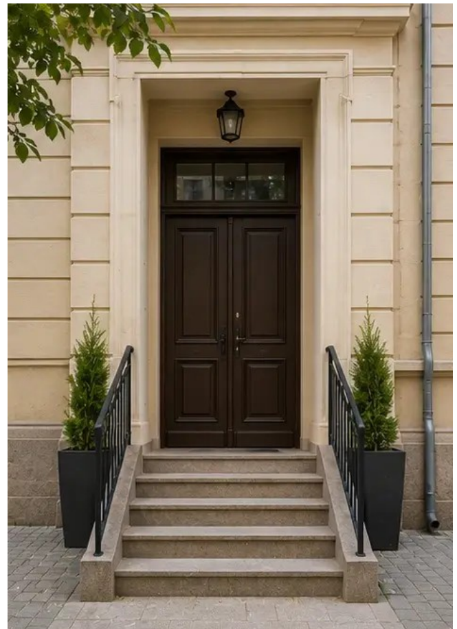
Foto №16 Property entrance after improvement
