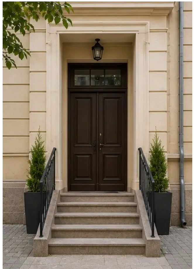
00 №16 Property entrance after improvement
