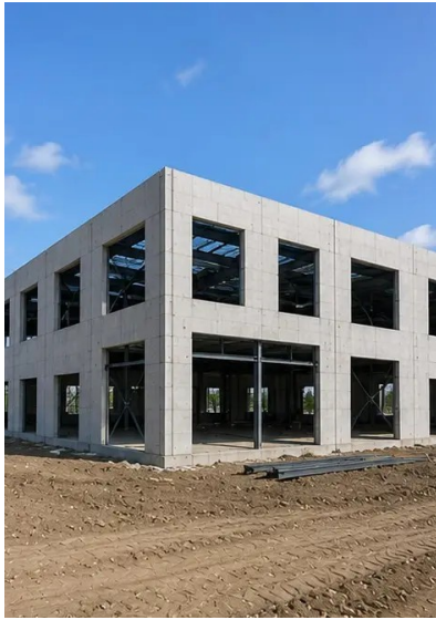
写真 №9. Structural frame completed according to project schedule
