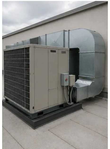
Photo #11. HVAC equipment condition assessed
