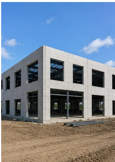
Fotó №9. Structural frame completed according to project schedule
