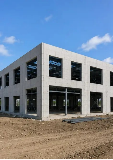
फोटो №9. Structural frame completed according to project schedule
