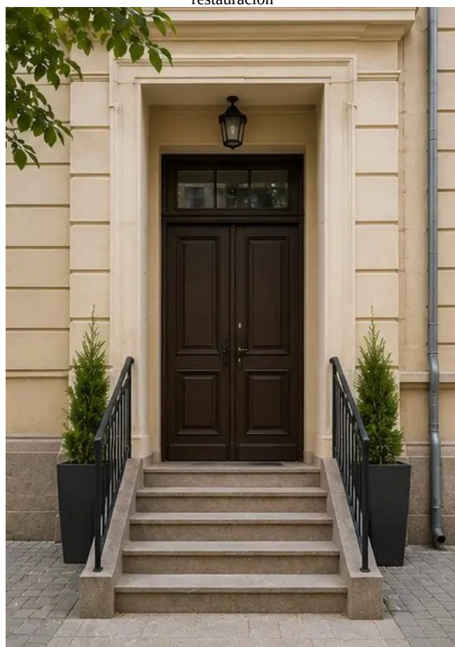
Foto №16 Property entrance after improvement
