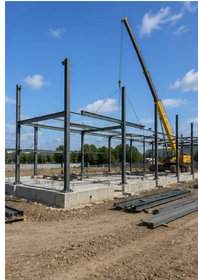
Photo #6. Structural frame assembly started
