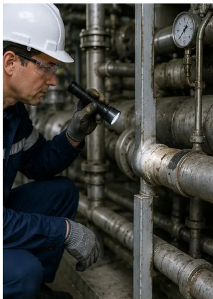
Photo #9. Pipe inspection completed according to maintenance schedule
