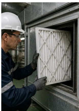
Photo #7. Air filter replacement completed
