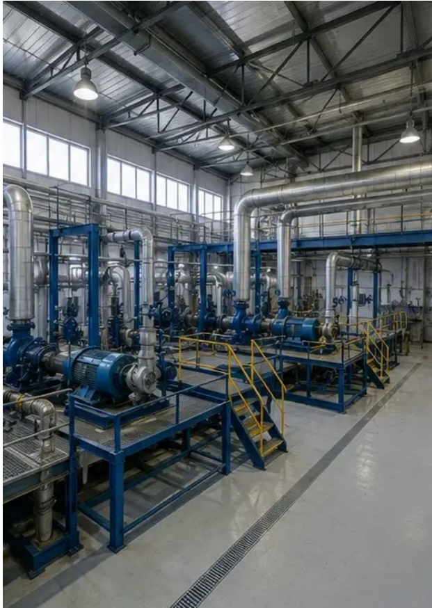
Photo #1. General overview of the industrial facility
