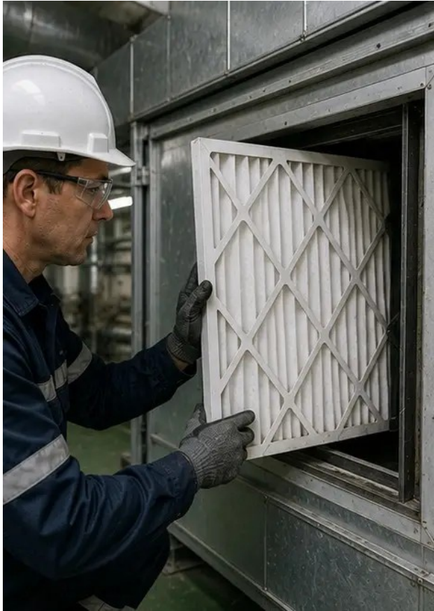
Photo #7. Air filter replacement completed
