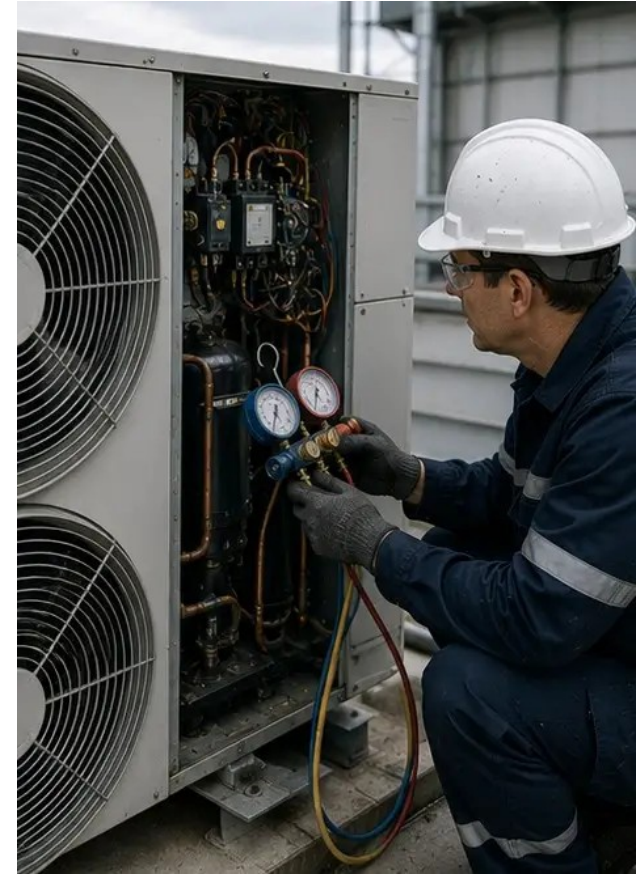
Photo #6. HVAC equipment condition documented
