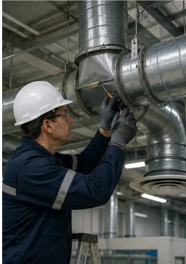
Photo #8. Ventilation system maintenance completed
