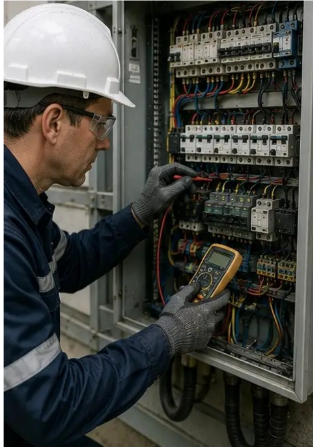
Photo #5. Electrical cabinet inspection performed
