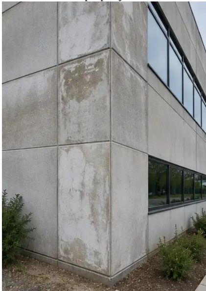
Photo #4. Exterior wall condition recorded during inspection
