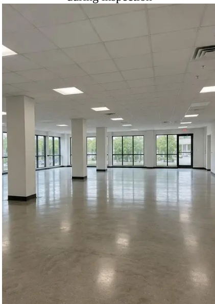
Photo #16. Final overview of the inspected property
