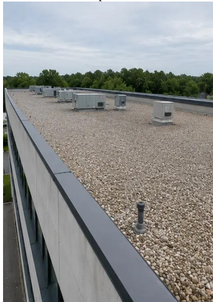
Photo #5. Roof condition inspection completed
