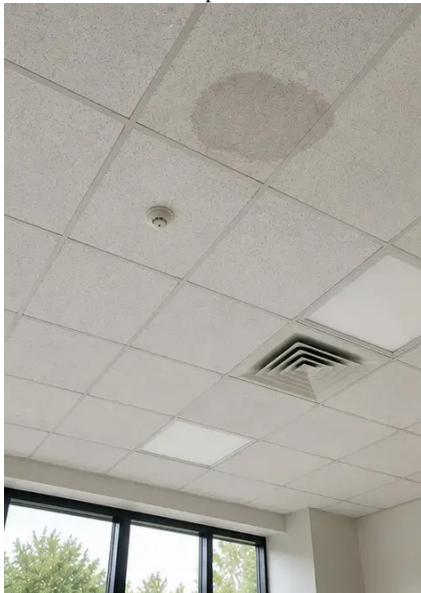
Photo #13. Ceiling condition documented during inspection
