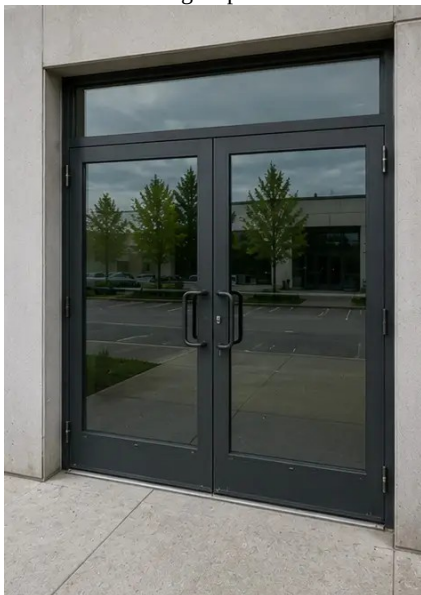
Photo #7. Door condition inspected and recorded
