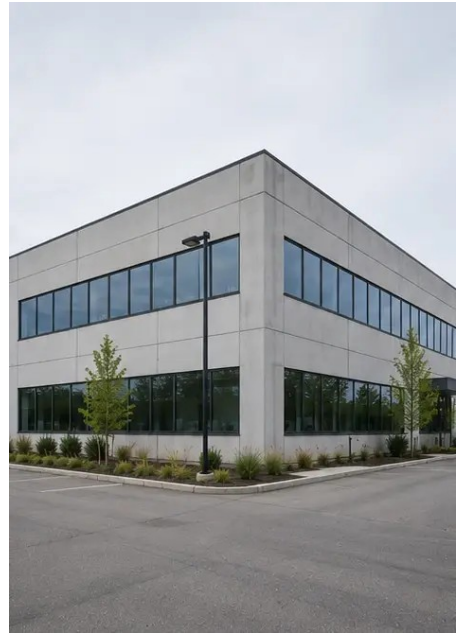
Photo #1. General view of the inspected property
