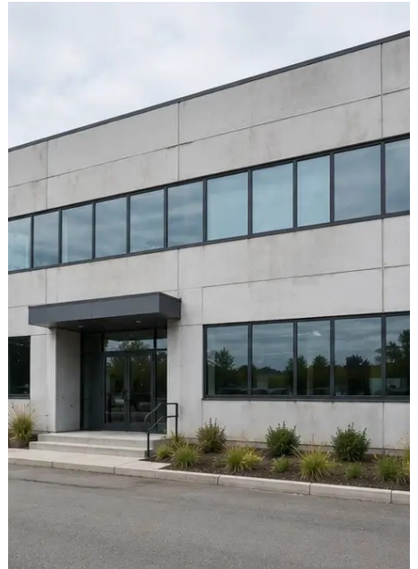
Photo #2. Front facade condition during inspection
