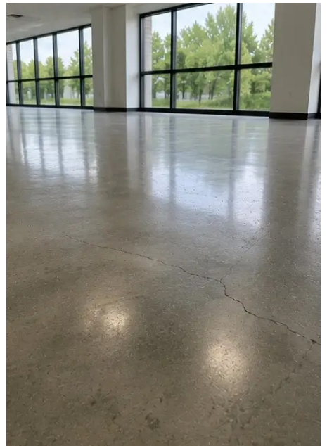
Photo #14. Floor condition assessed and recorded
