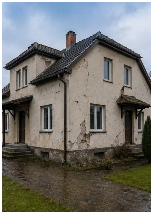
Photo #1. General view of the inspected property
