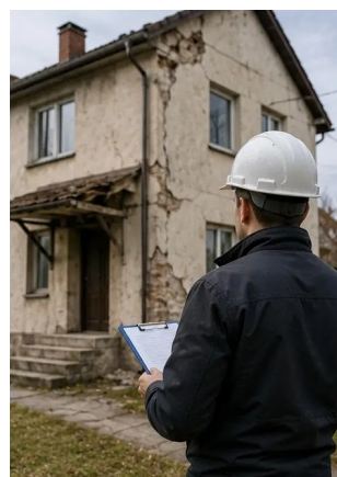
Photo #16. Final damage inspection summary photograph
