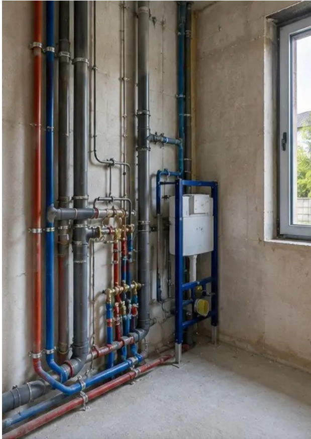
Photo #10 Plumbing systems installation completed in designated areas
