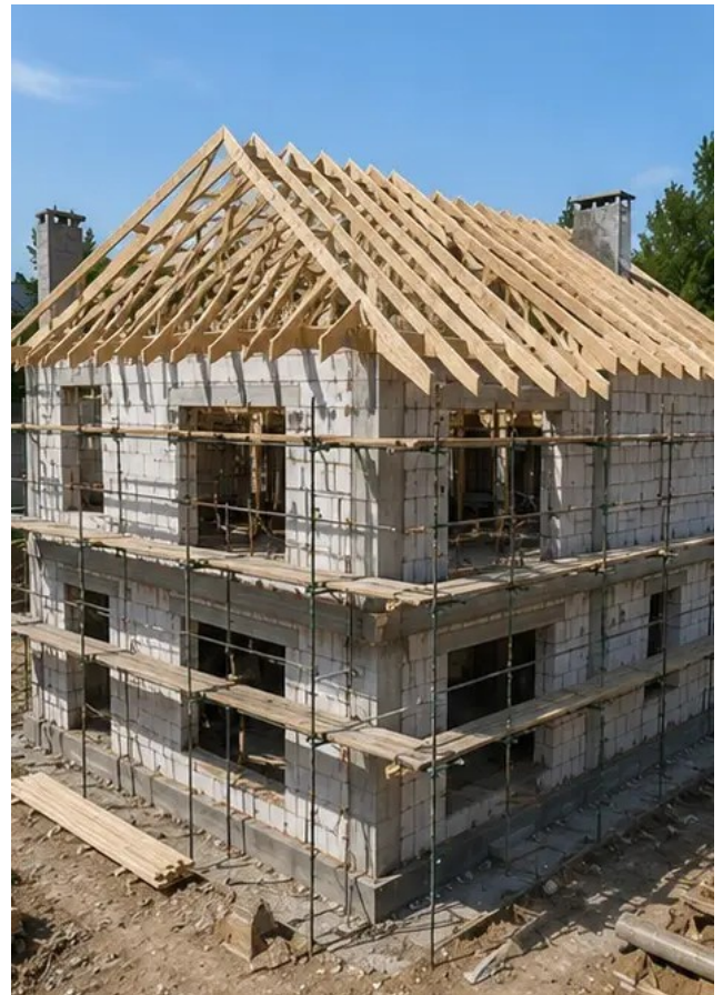
Photo #8 Roof installation work completed
