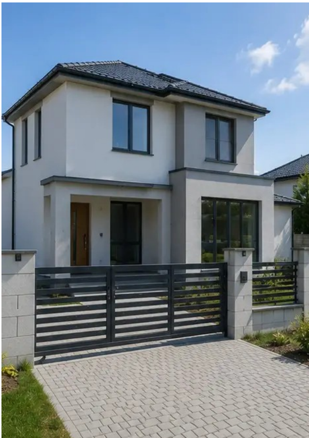
Photo #15 Completed building exterior after construction
