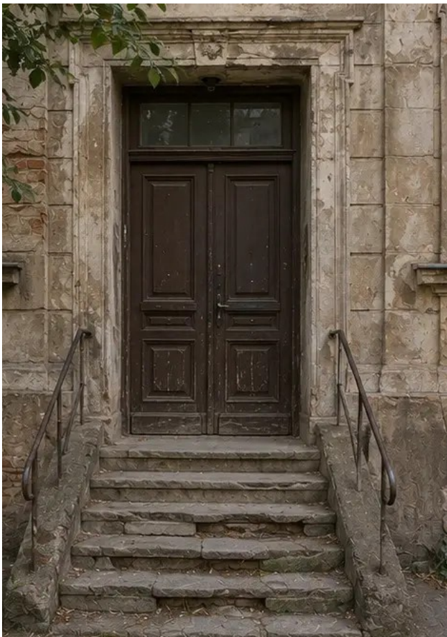
Photo #15 Property entrance before improvement
