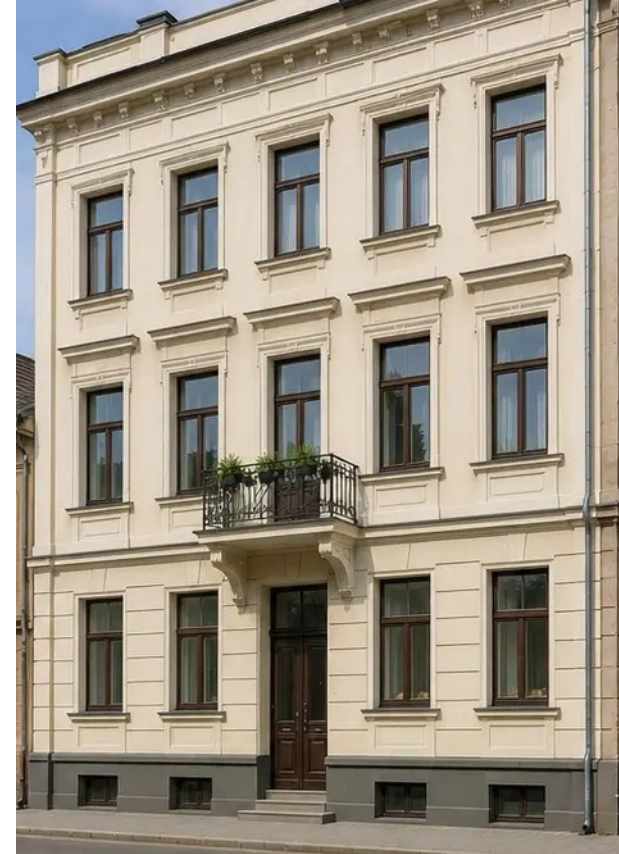
Photo #14 Building facade after restoration work
