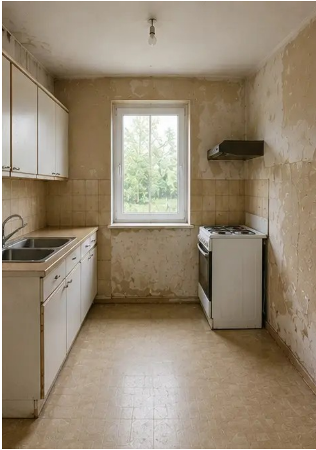
Photo #11 Kitchen condition before renovation
