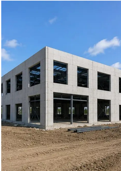
Foto №9. Structural frame completed according to project schedule
