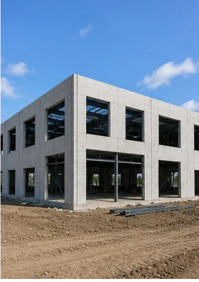
ফটো নং৯. Structural frame completed according to project schedule
